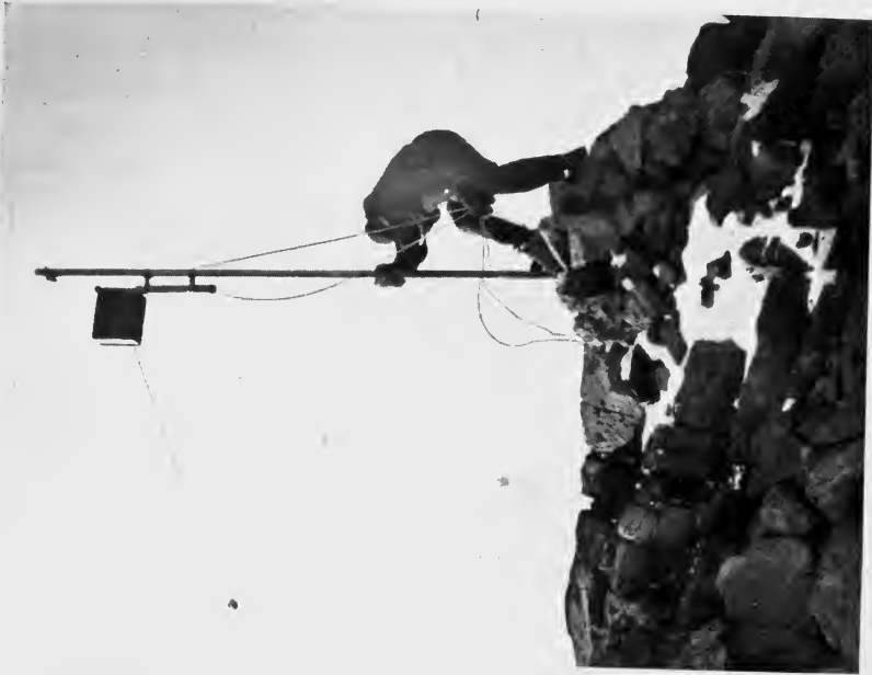
Adelie Land THE PUFFOMETER, DESIGNED TO RECORD HURLEY MAXIMUM GUST VELOCITIES
